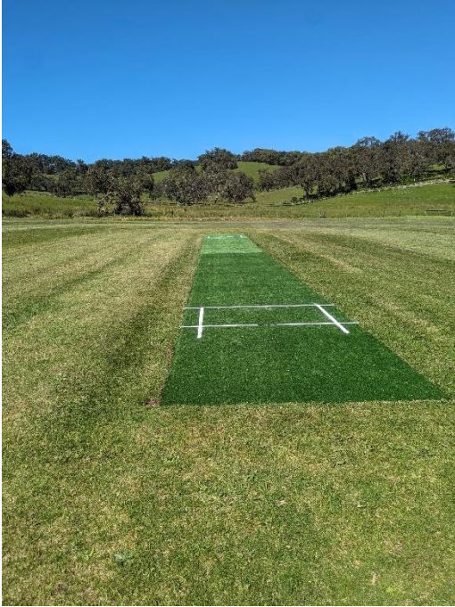
Hoddles Creek Cricket Club - Pitch Repairs
