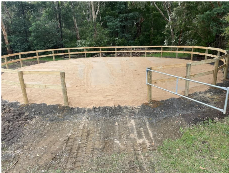
Upper Yarra Pony Club - Leveling, fencing and surfacing of round yard
